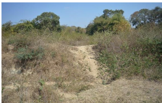
Figure 6. Breakage on EPT
